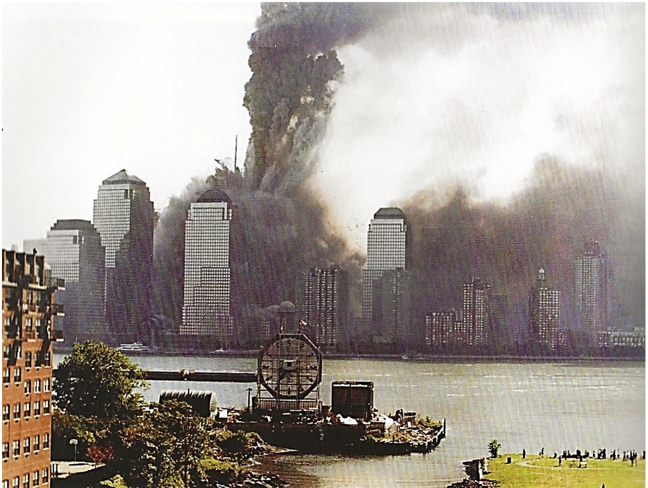
Fingers of lather emerge upward as North Tower collapses
